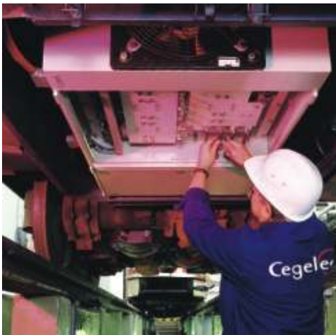
Assembly of TV Progress traction equipment
