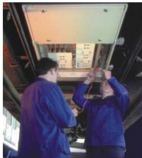
Assembly of TV Progress traction equipment
